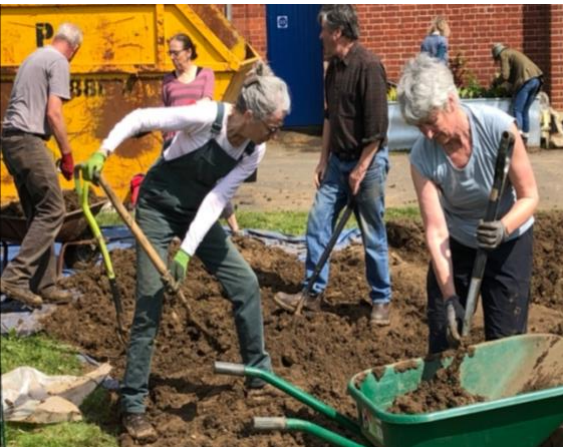
Making the rain garden bed, May 2024
