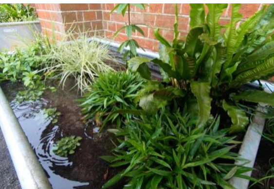
Rain from the roof flows into planted trough, May 2024
